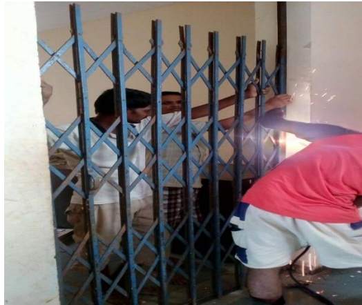
Making an iron grill type partition for the store room
